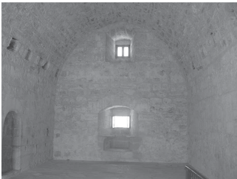
Fig. 83: Kolossi, keep, middle storey, eastern room, looking west [M. Olympios].
